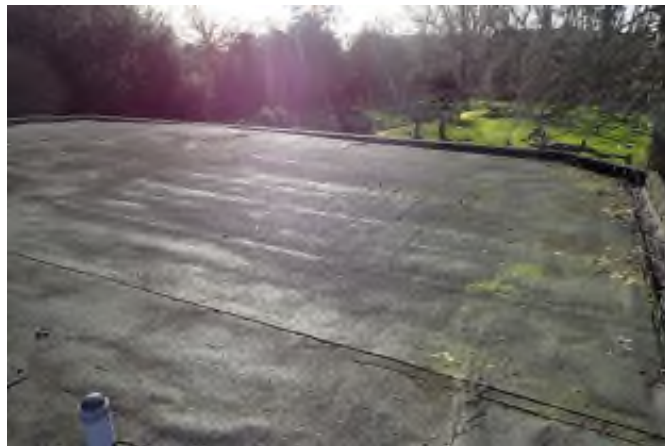
Church Hall Roof
